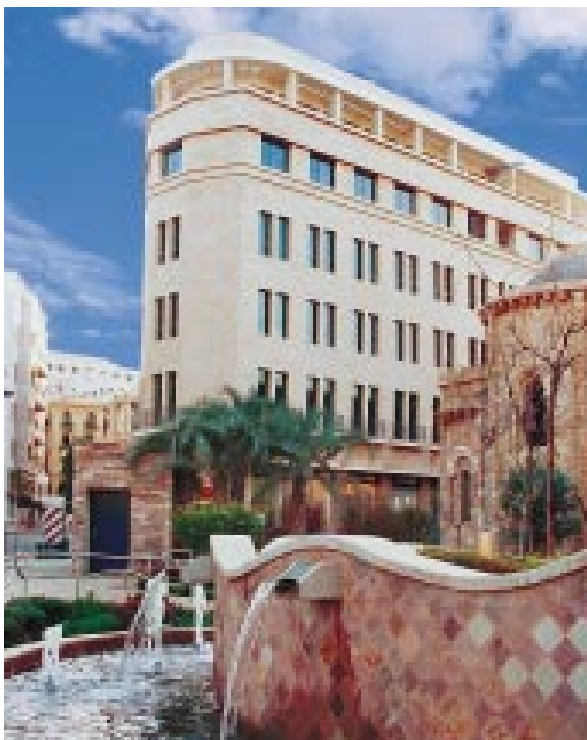
Lot 200 office building.
