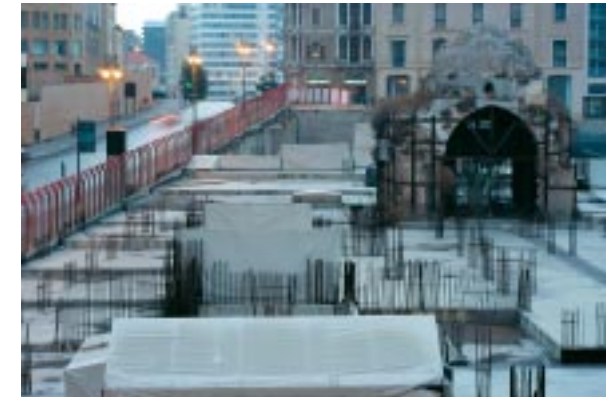
Souks of Beirut: south Souks site along Weygand street.
