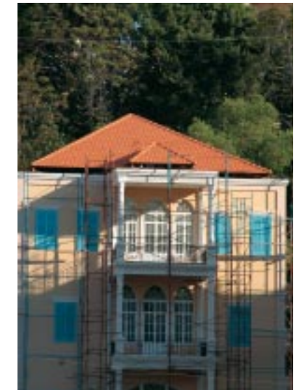
Lots 800 and 802 under restoration.
