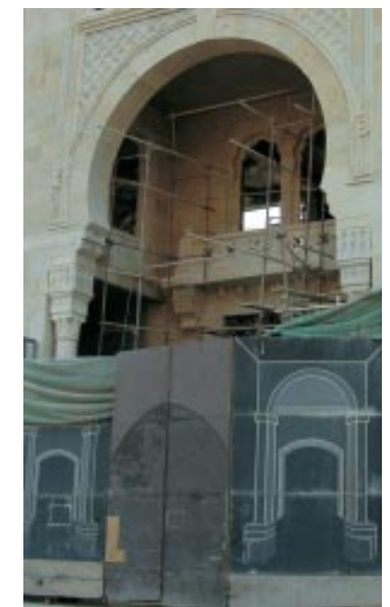
Stone repairs on the Grand Theatre façades.
